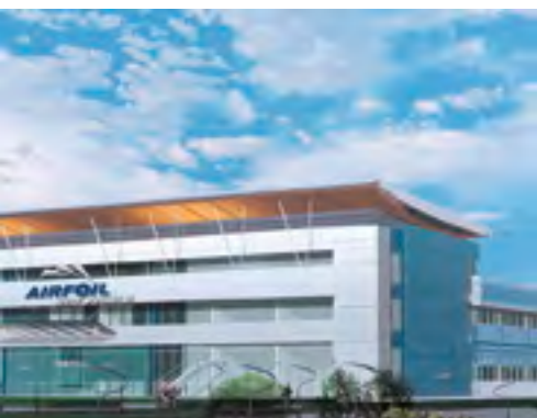
The ASSB blade repair shop in Malaysia.
