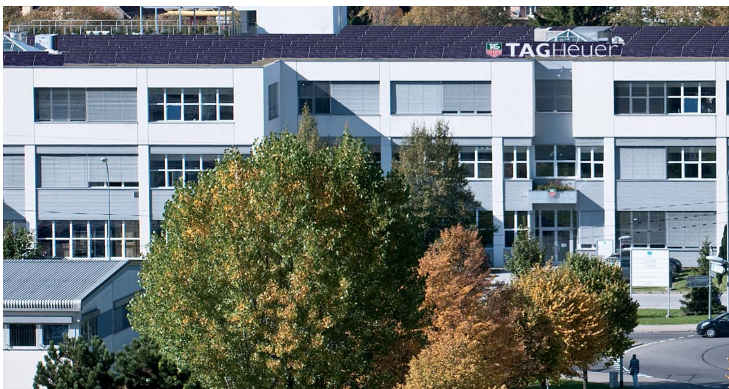
TAG Heuer is installing 750 m2 of photovoltaic panels on the roofs of its buildings in La Chaux-de-Fonds.
